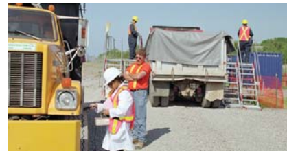
Trucks are monitored for radiation and securely covered before transporting waste.
